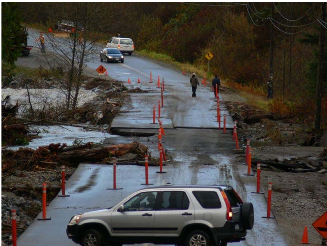
Flooding of Chilliwack Lake Road, November 2006.
