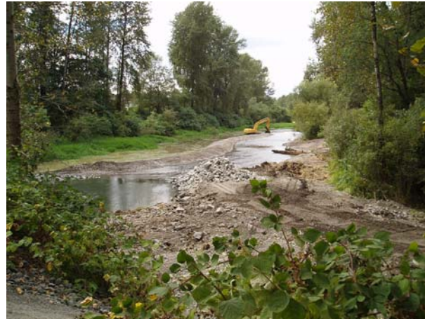
Getting close to completion...
