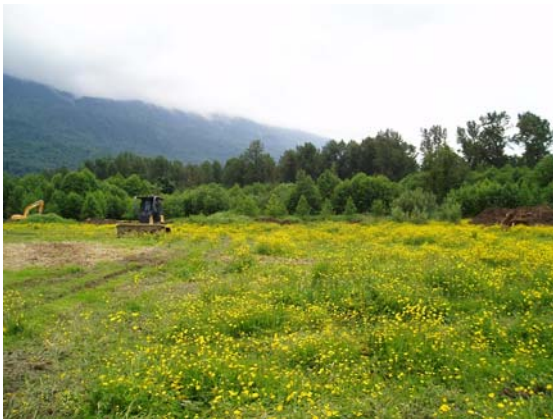
Early stages of construction at Salwein Creek
