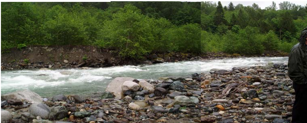
The far bank is where groynes will be placed using boulders from the abandoned side channel
