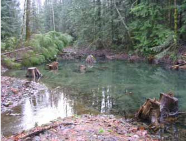
Newly constructed ponds at Thompson Park.
